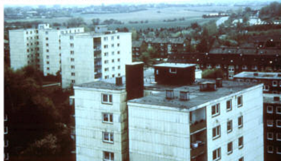
Blocks towers before renovation
