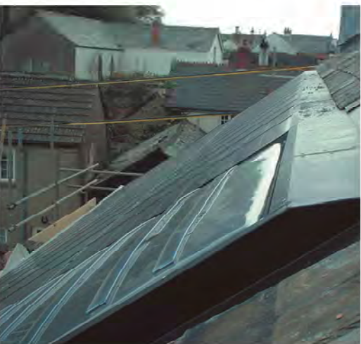
Twin heating collectors with 1 kWp PV
