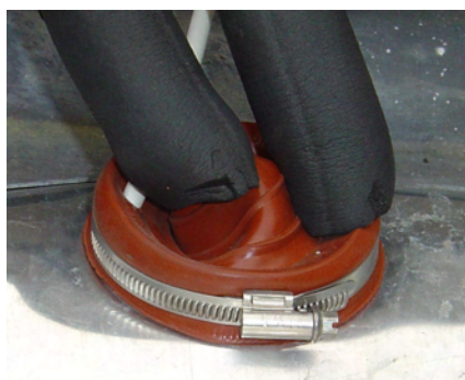
A3 Figure 1: Photo of optional aluminium flashing supplied by ISL
