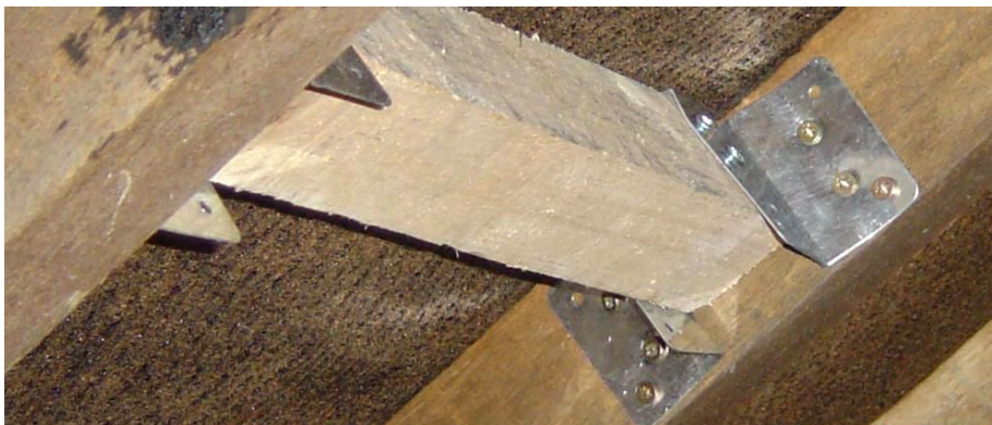
Photo of noggings in roof space to fix frame to
